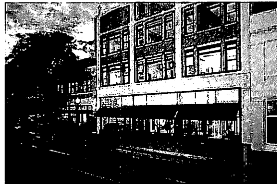
Corporate Headquarters, Sumter, SC
